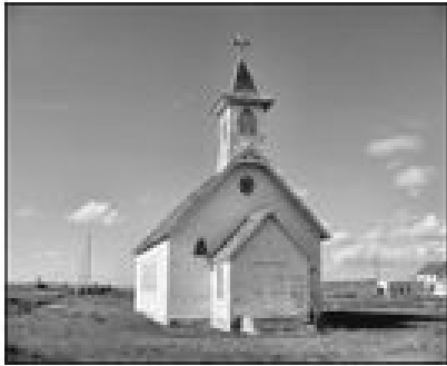
Christ Church Episcopal Restored 1800's Church
