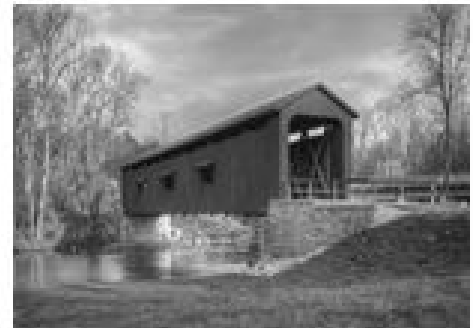
Pass Thru Covered Bridge
