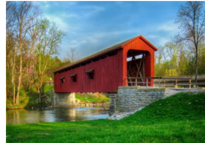
Pass Thru Covered Bridge
