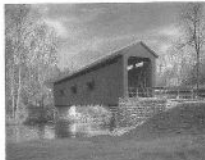
Pass Through Covered Bridge
